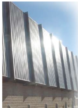
Solar panels being tested on Walmart store
